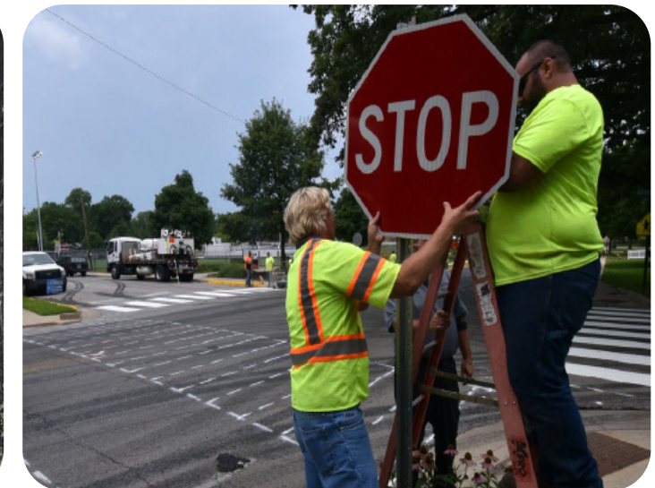
Photo: Installation of Stop Sign
