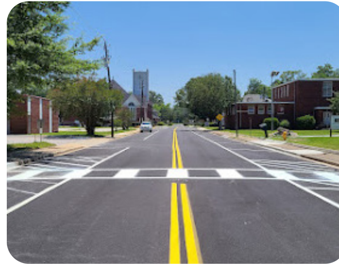
Photo: Resurfacing and striping on Council St.
