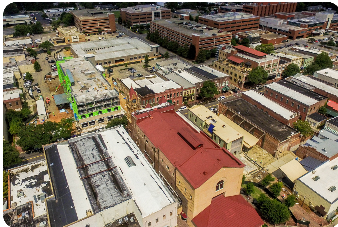
Photo: Construction in Downtown Sumter
