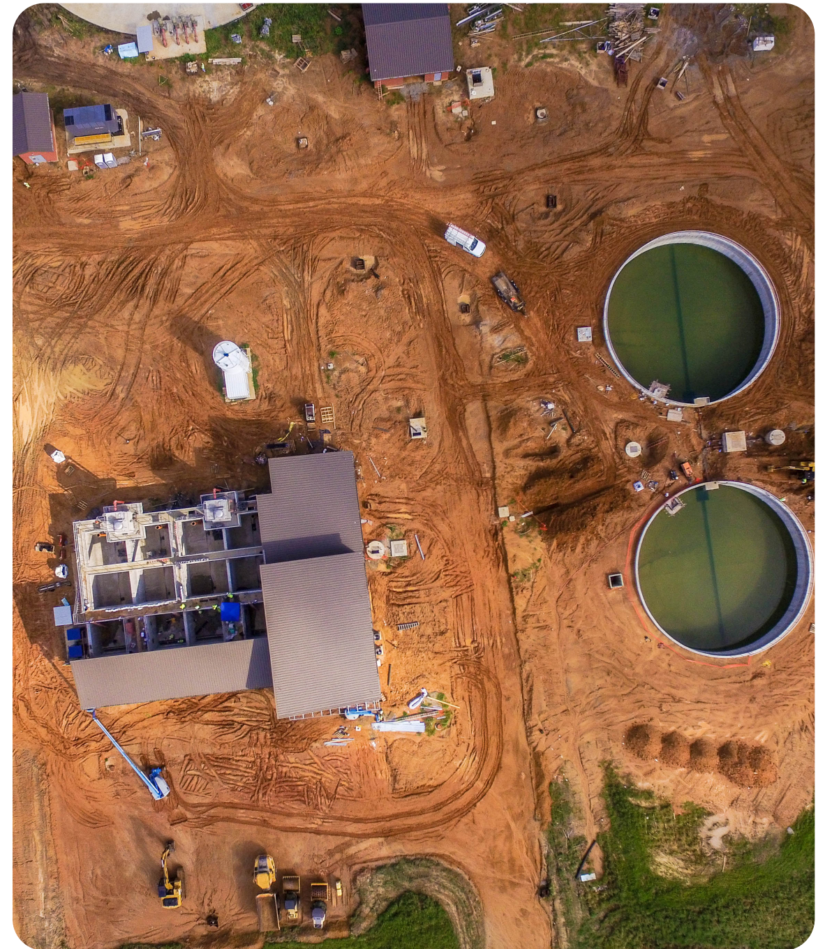
Photo: Construction of Wastewater Treatment Plant #6
