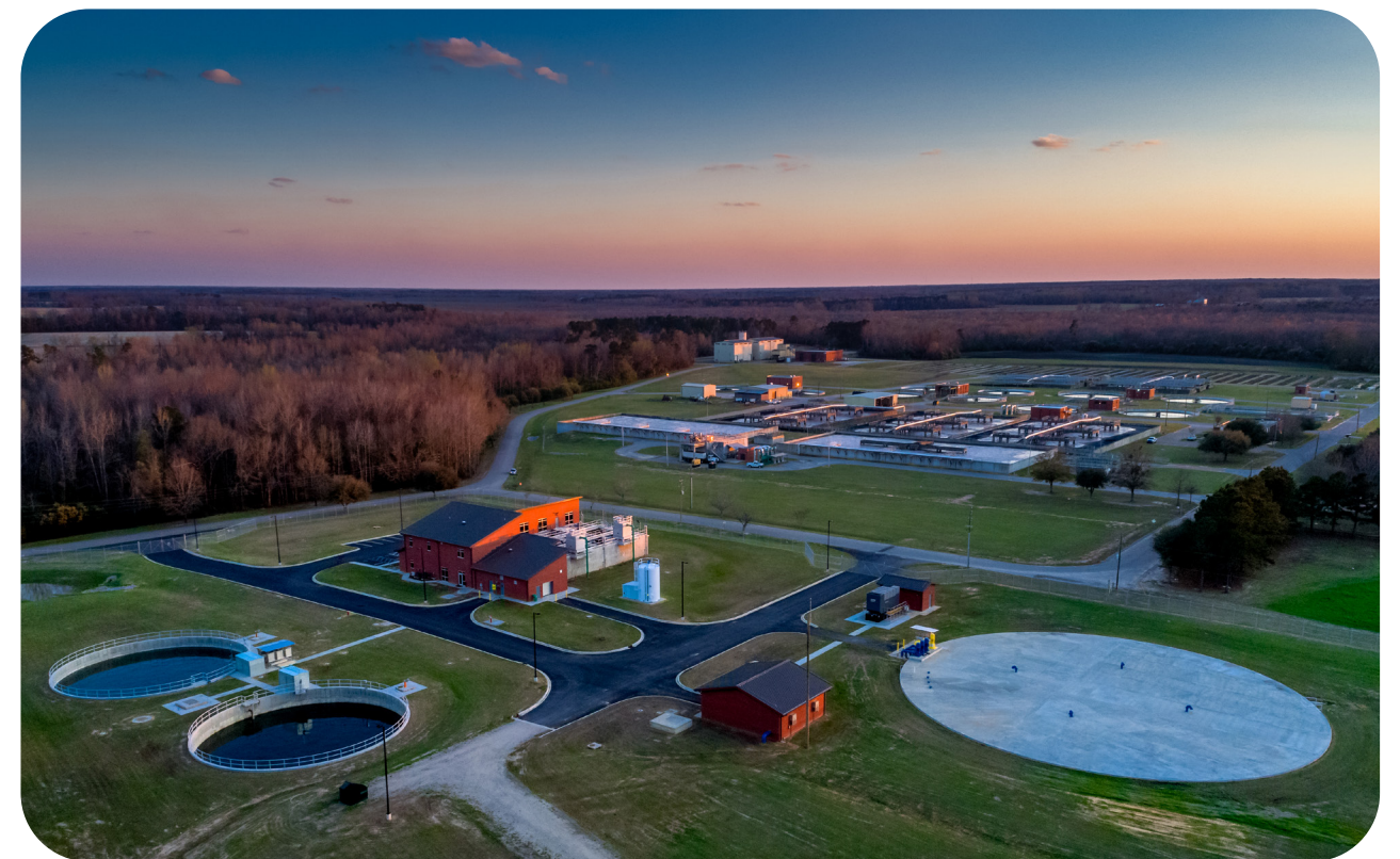
Photo: City of Sumter Wastewater Treatment Plant #6
