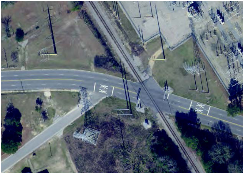
Rail Crossing at East Red Bay Rd.
