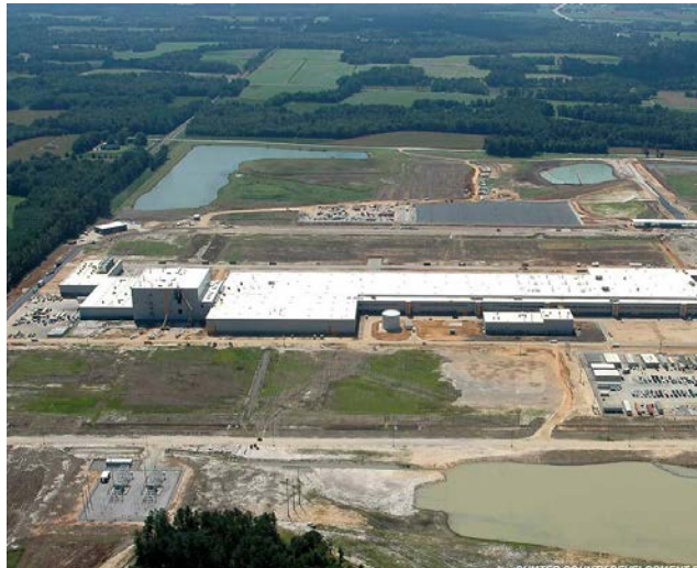
AERIAL IMAGE OF CONTINENTAL TIRE'S $500 MILLION MANUFACTURING FACILITY UNDER CONSTRUCTION, 2013
