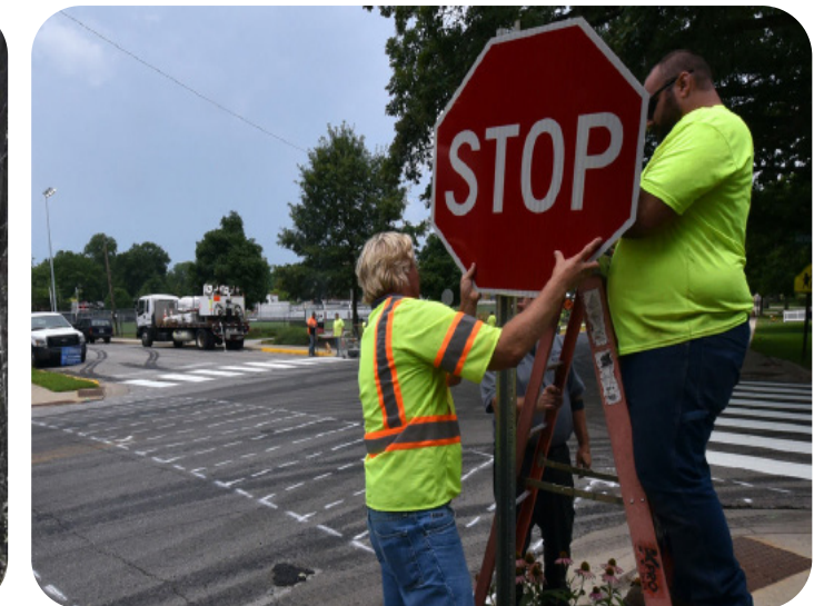
Photo: Installation of Stop Sign
