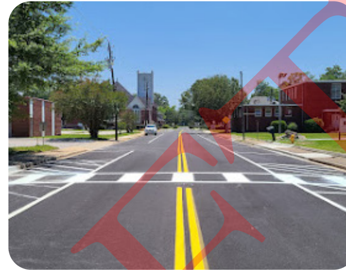
Photo: Resurfacing and striping on Council St.
