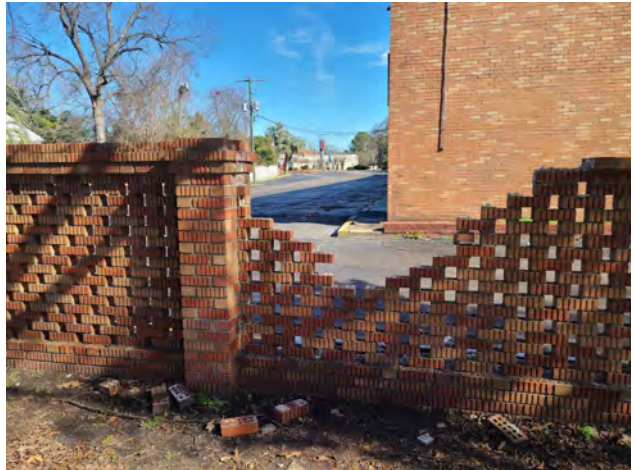
Above Right: Existing Brick Wall/Fence on north, west, and south property lines (only damaged section shown)
