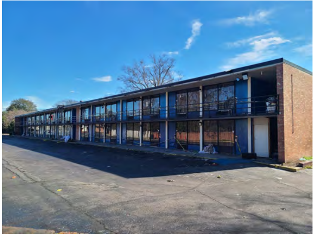
Above Left: Motel building as viewed from northwest corner of property (Church St. ROW)
