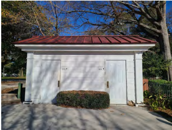
Above: Existing park restroom building (front view)
