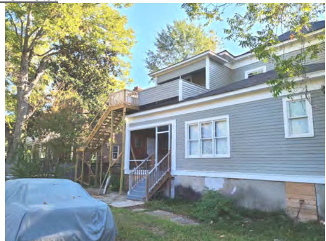
Rear Façade, as viewed from southwest corner of lot, showing area of proposed alteration.
