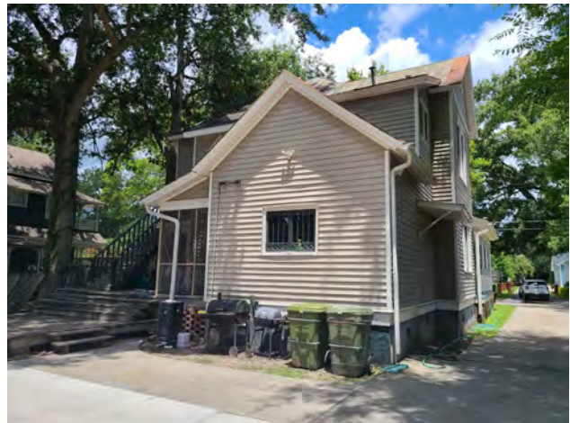
Rear Façade, as viewed from southeast corner of lot
