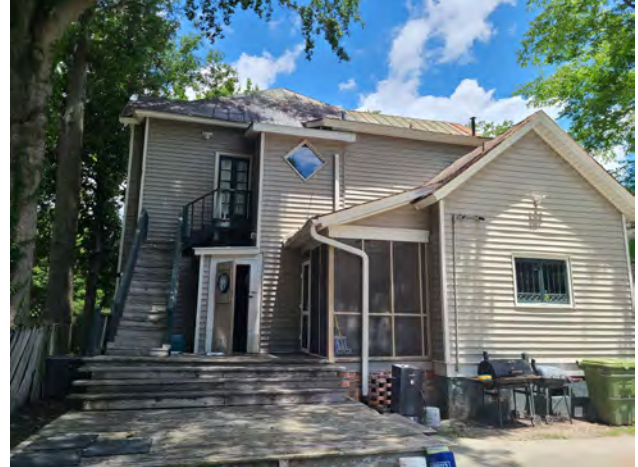
Rear Façade, as viewed from southwest corner of lot
