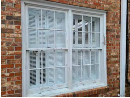
Example of paired 6 over 6 double hung wood window found on rear façade
