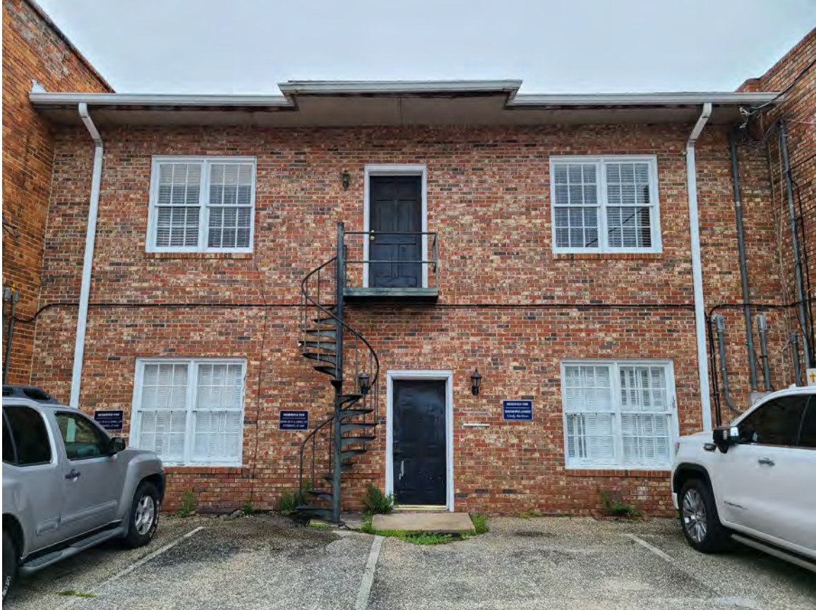
Above: Current building rear exterior, viewed from parking lot.
