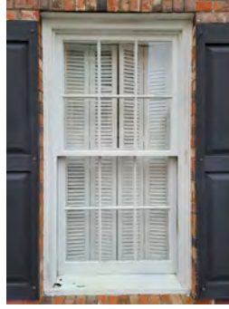
Example of 6 over 6 double hung wood window on front façade
