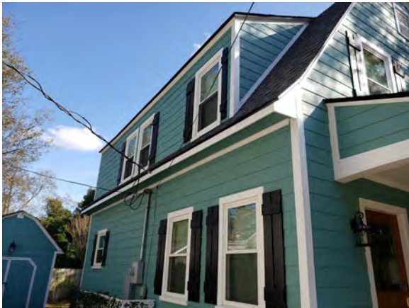
North-facing Exterior (proposed for gutter installation)
