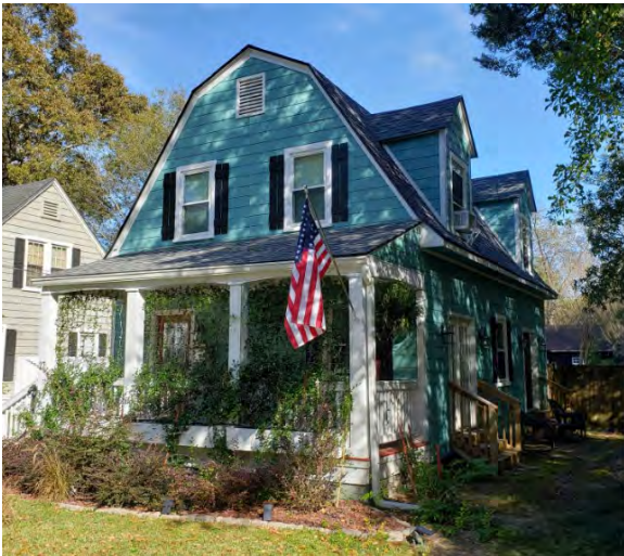
Front Façade (pre-renovation)
