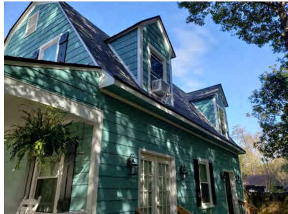
South-facing Exterior (proposed for gutter installation)
