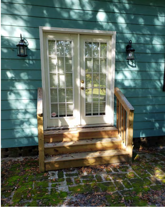
South-facing East Exterior Steps
