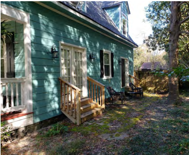
South face of building (site of proposed deck and stair reorientation)
