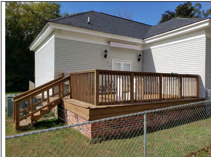
Existing Deck (Site of proposed screen porch)
