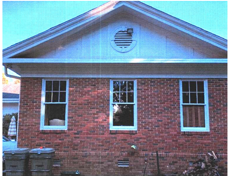
Existing rear of structure (facing view)
