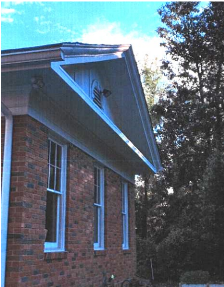
Existing rear of structure (side view)
