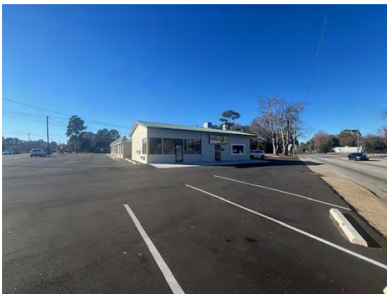
Above: Picture of 667 W. Liberty St. Building
