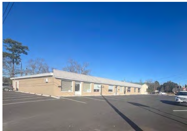
Above: Picture of 669-675 W. Liberty St. Building
