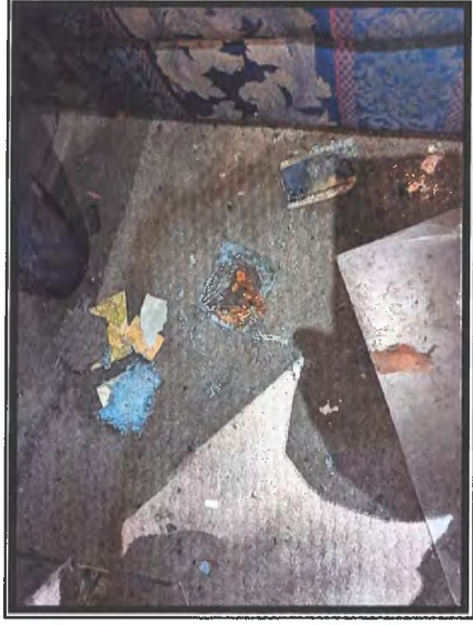
Photo #6 No Asbestos Detected in Carpet Layers
