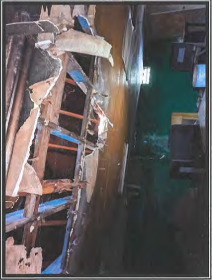
Photo #9 No Asbestos Detected in Sheetrock System of the West Section
