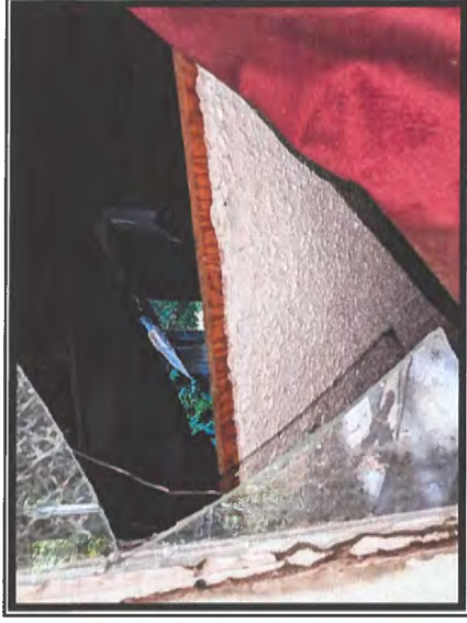
Photo #6 View Depicting Plywood Ceiling Panel with Spray-applied Texture
