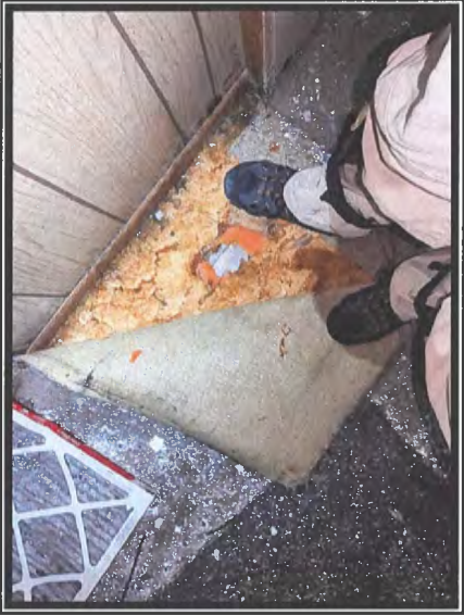
Photo #9 No Asbestos Detected in Carpet Materials
