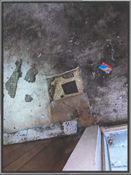
Photo #9 No Asbestos Detected in Tan Weave-design Sheet Flooring under Carpet
