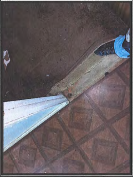
Photo #5 No Asbestos Detected in Any Resilient Flooring or Carpet Layers
