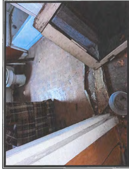
Photo #2 Asbestos Detected at 3% in Sheetrock Ceiling System
