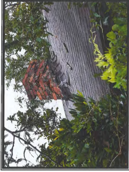
Photo #2 Chimney Sealant Material is Presumed to Contain Asbestos
