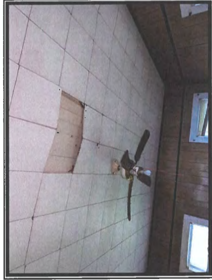
Photo #7 No Asbestos Detected in Cellulose-based Ceiling Tiles in Room 112B
