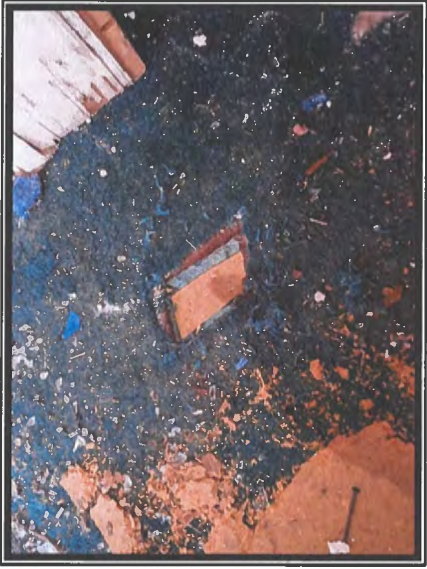
Photo #5 No Asbestos Detected in Any Floor Covering Layers
