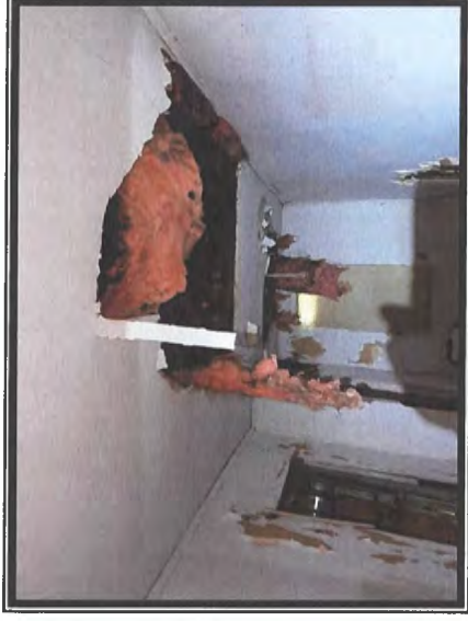
Photo #6 No Asbestos Detected in Sheetrock Ceiling and Wall System
