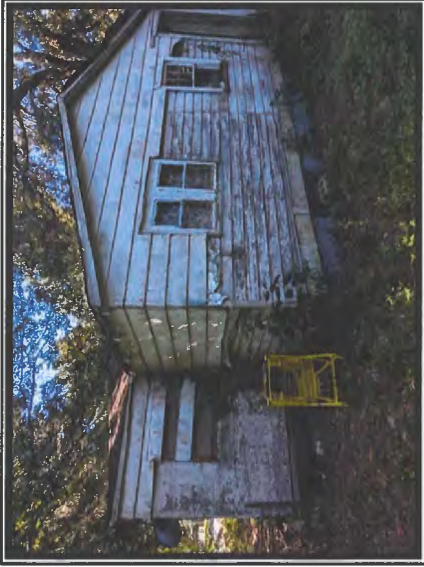
Photo #1 View Depicting Wood Slat and Fiberboard Plank Exterior Siding
