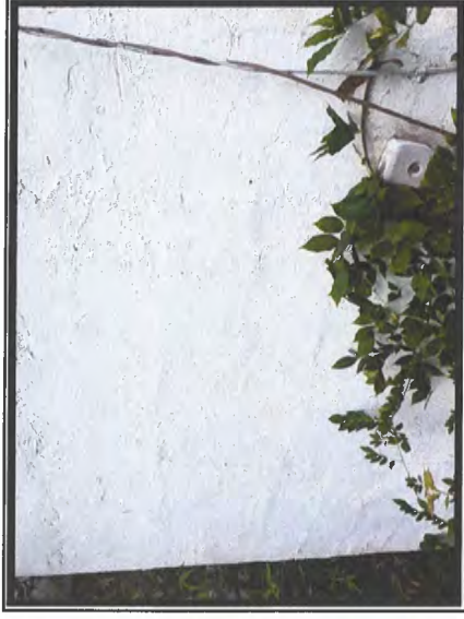
Photo #2 No Asbestos Detected in Exterior Wall Surfacing Material
