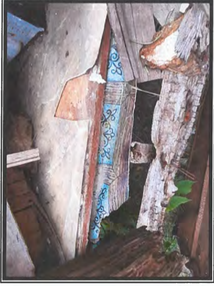
Photo #6 No Asbestos Detected in Tan-colored or Green and Brown-colored Sheet Flooring
