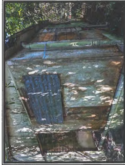
View Depicting Asbestos-containing Roofing Material on Collapsed Stoop Feature
