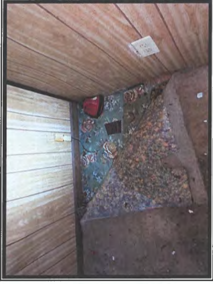
Photo #10 No Asbestos Detected in Green Floral-design Sheet Flooring under Carpet
