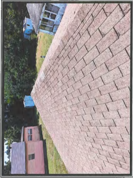
Photo #6 No Asbestos Detected in Roofing Shingles or Associated Felt Material
