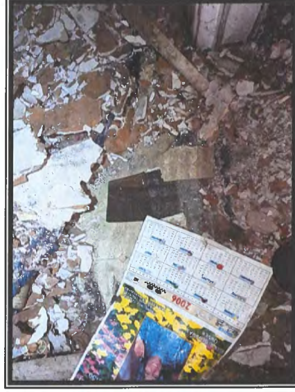
Photo #6 No Asbestos Detected in Sheetrock with Joint Compound Ceiling System
