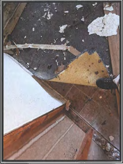
Photo #5 No Asbestos Detected in Carpet or Sheet Flooring Materials
