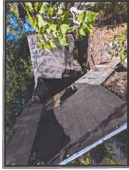
Photo #2 No Asbestos Detected in Exterior Fiberboard Wall Panels or Sheathing Board
