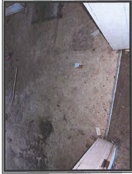
Photo #11 No Asbestos Detected in Tan Square-design Sheet Flooring
