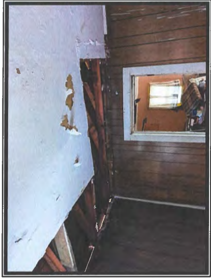
Photo #2 Asbestos Detected at 3% in Sheetrock Ceiling System
