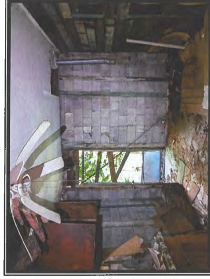
Photo #6 No Asbestos Detected in Sheetrock Ceiling and Wall System
